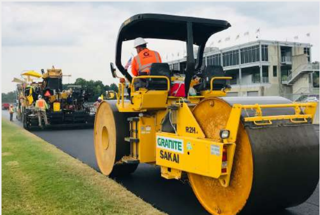
Granite Construction has referred to the R2H-4 as their “secret weapon” to achieve notable smoothness on racetrack jobs such as this repave of historic Barber Motorsports Park in Birmingham, AL.
