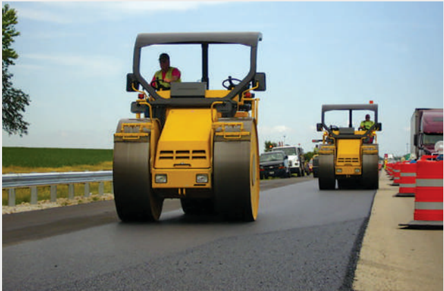
Two R2H-4 three wheel static rollers run in echelon formation
